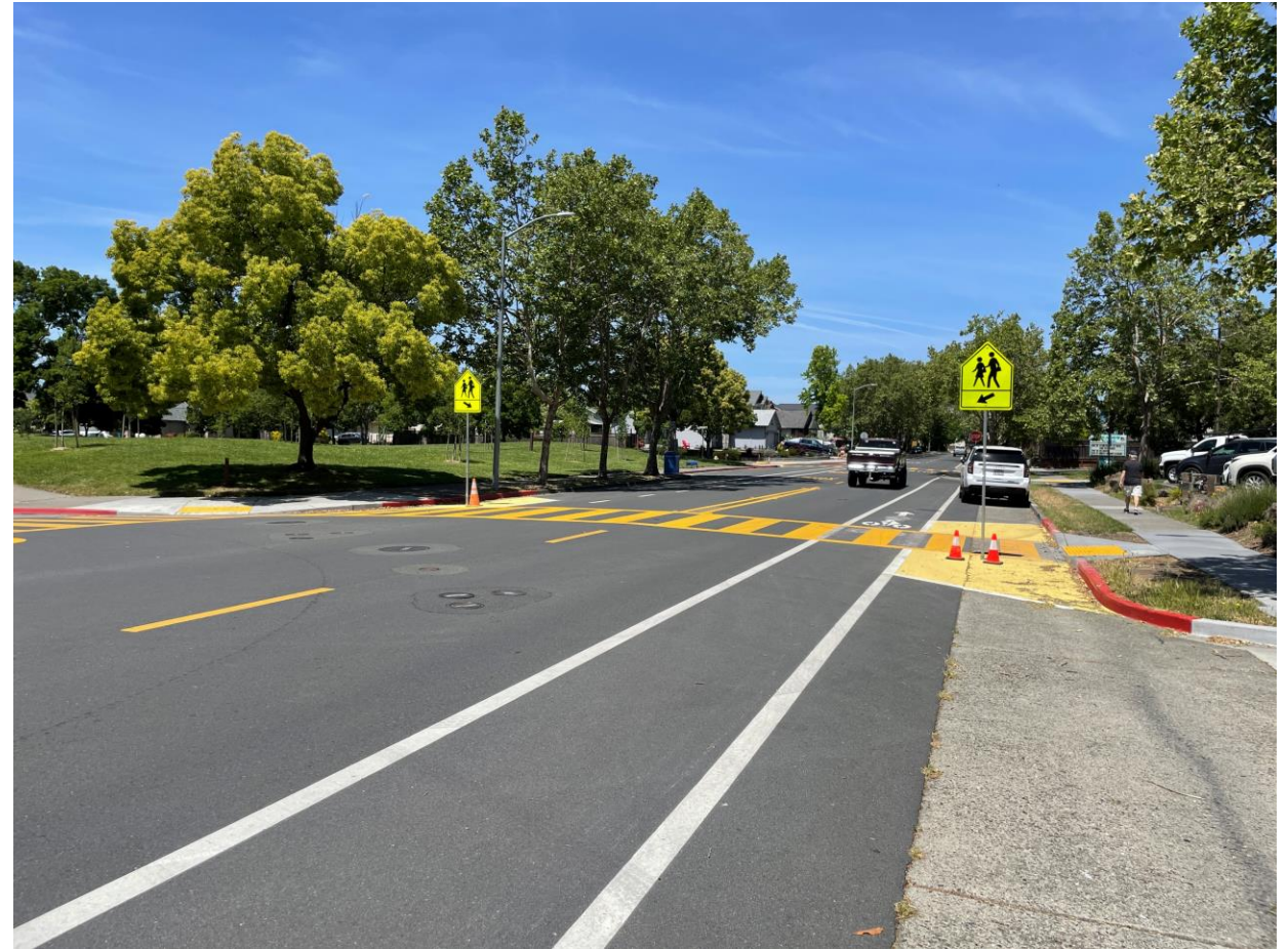
Bulbout & New Crosswalk at Maria Drive & Yarberry Drive (Meadow)
