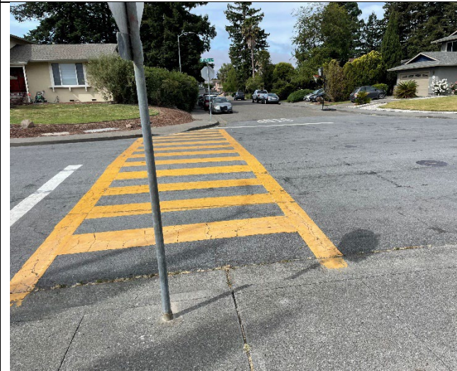
Crinella Drive & Filippini Way crosswalk – add curb ramp at the entrance to the Crinella Drive pocket park
