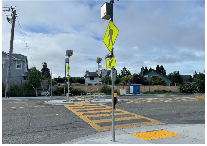
Uncontrolled crossing with median and flashing beacons on Casa Grande Rd. in front of school driveway loop
