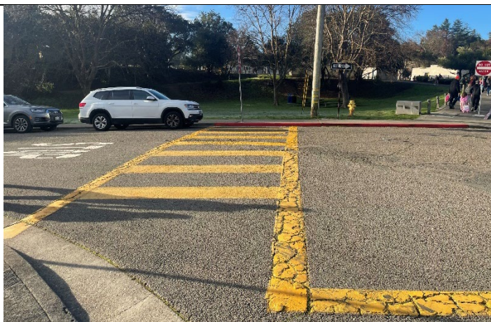
Eastern leg of crosswalk across Cherry St. at Antone Way. No curb cuts on the south side, curb cut on north side is not ADA compliant and is not aligned with marked crosswalk.
