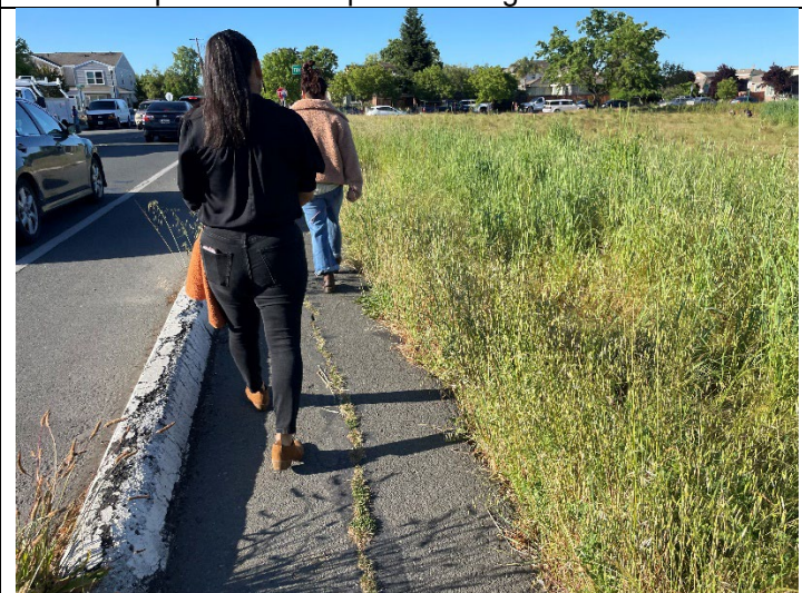
Berm is fairly narrow, in poor condition, and often overgrown with weeds (property owner responsibility)
