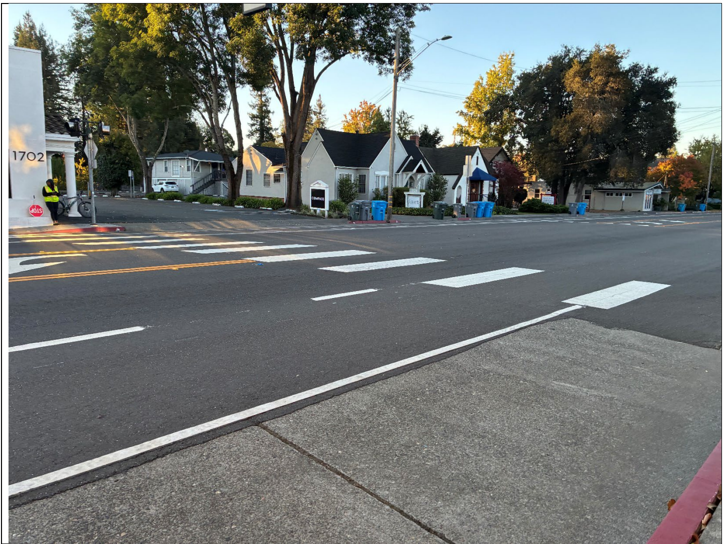
Monitored crosswalk at 4 th St. and Proctor Drive (consider relocating Crossing Guard to Talbot Way instead)
