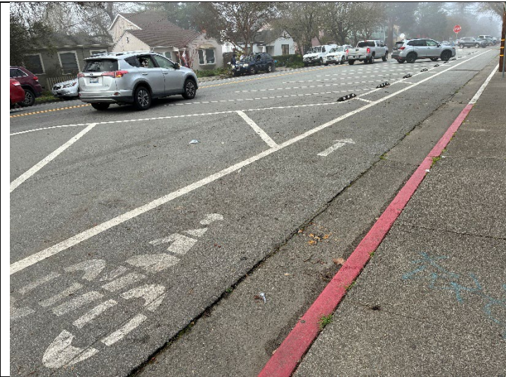
Parking protected bike lane between student parking lot and Armory Drive (consider extending bike lane to Mendocino)
