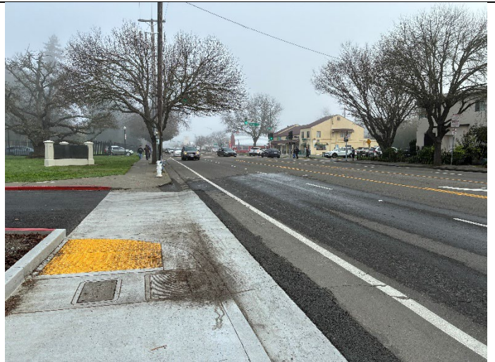
School district: consider marking crosswalks across school driveway entrances and exits
