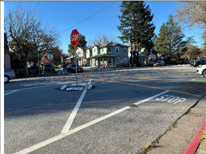
Drivers "cut corner" at Glenn St. & Ridgway and maneuver around this stop sign – add delineators to prevent
