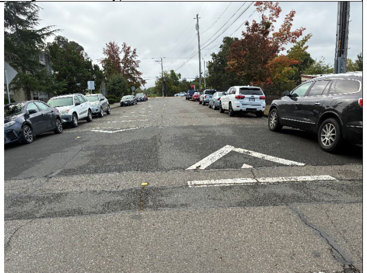
2 nd speed hump on Jack London Drive, closer to Hwy 12 (convert to raised crosswalk?)
