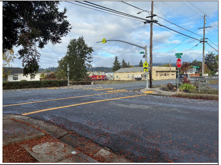
Intersection of Middle Rincon Road and School Street – recently installed RRFB; bike lanes would be beneficial on Middle Rincon Road
