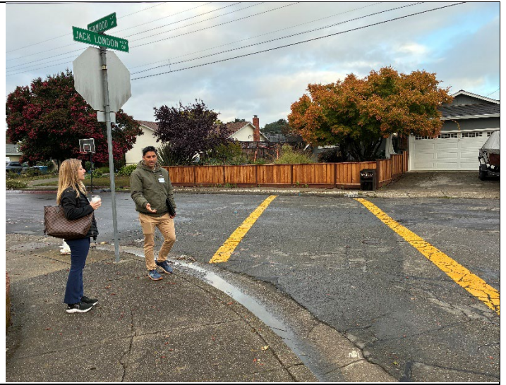
Intersection of Jack London Drive and Rinwood Drive – needs curb ramps, consider curb extensions
